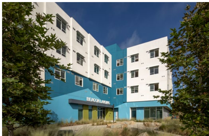
Completed construction of Beacon Landing
