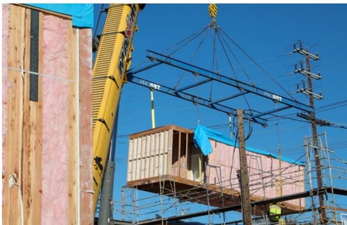
Modular construction of Beacon Landing
