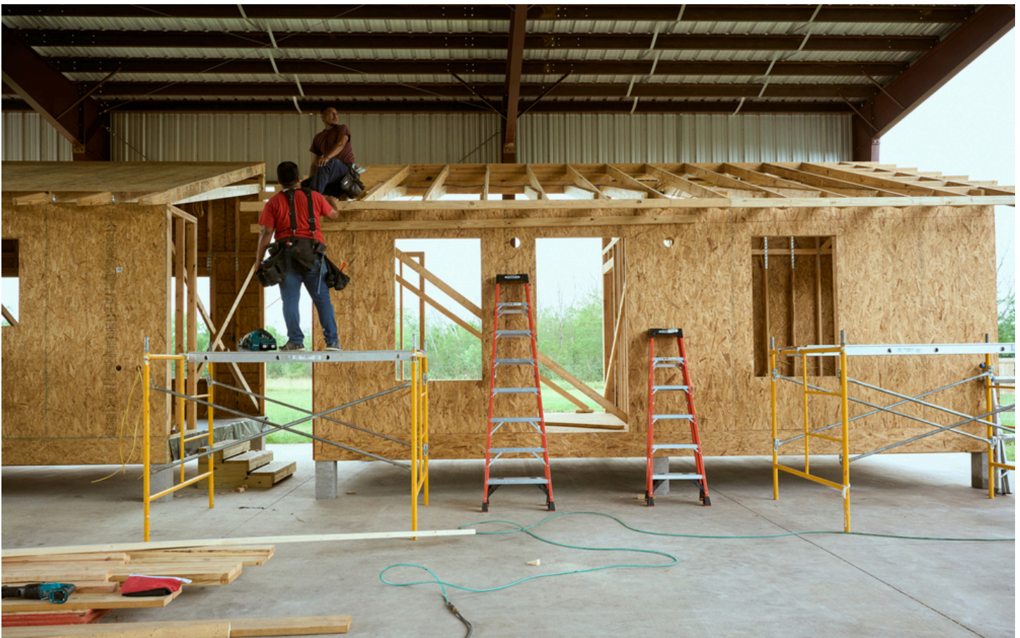
DreamBuild homes under construction at The Farm, an off-site manufacturing facility, in Los Fresnos, Texas.
