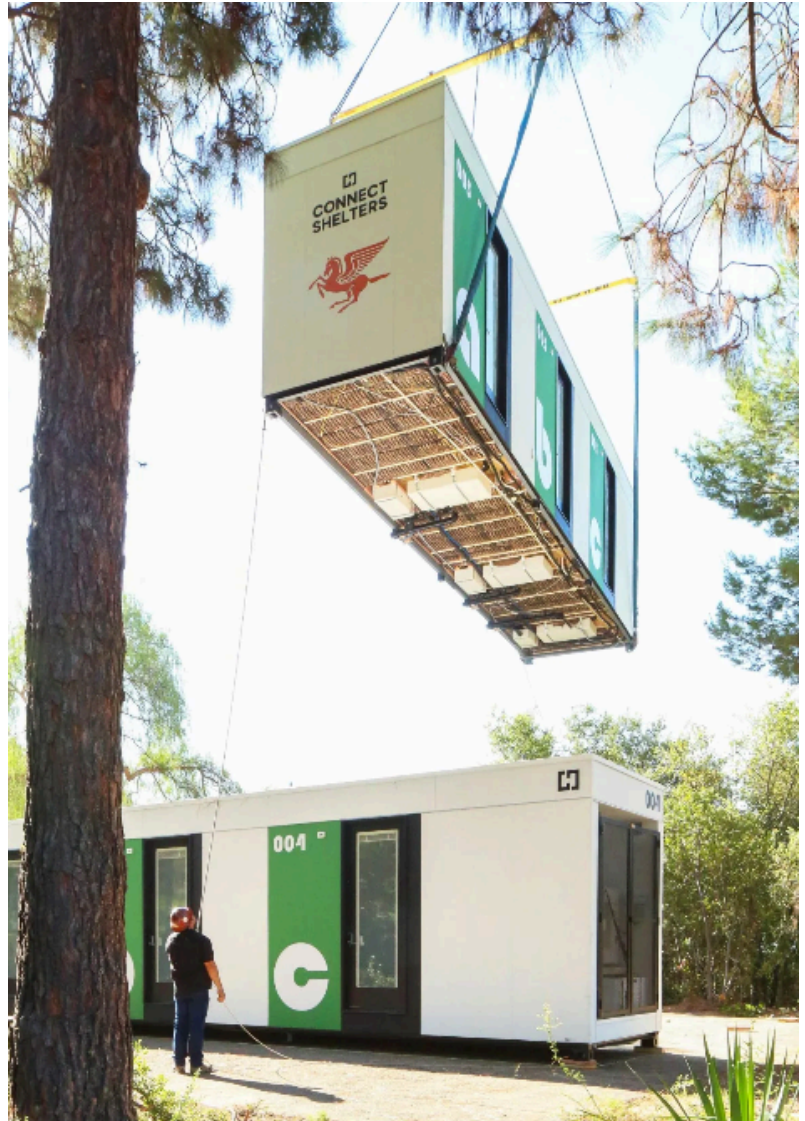
Connect Shelter unit lifted by crane
