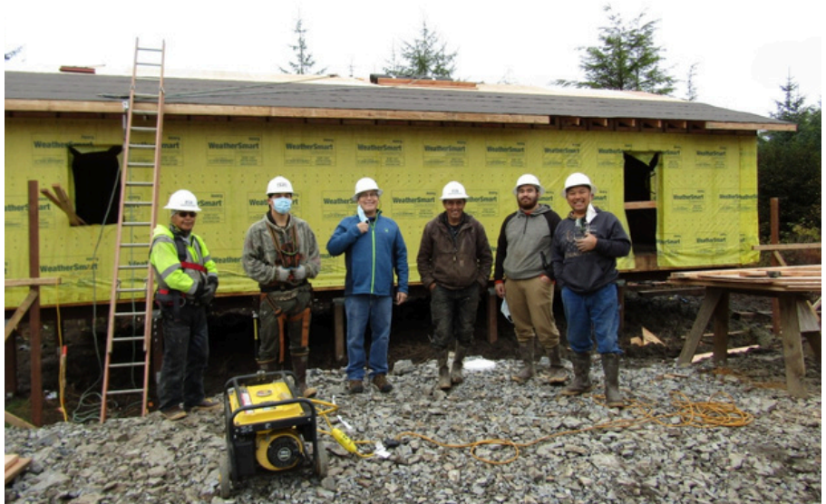
A local construction crew builds a new home through Success Starts with Me in Angoon, Alaska.
